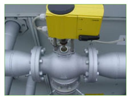
The 3-way-valve is an control arrangement which:
