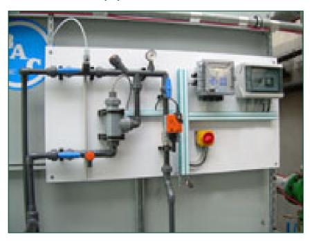
BAC offers a wide range of **automatic water treatment packages** to control corrosion, scaling, fouling and microbiological growth in cooling systems incorporating BAC condensers.
