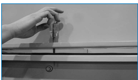
Usage of drift pin to align the screw holes
